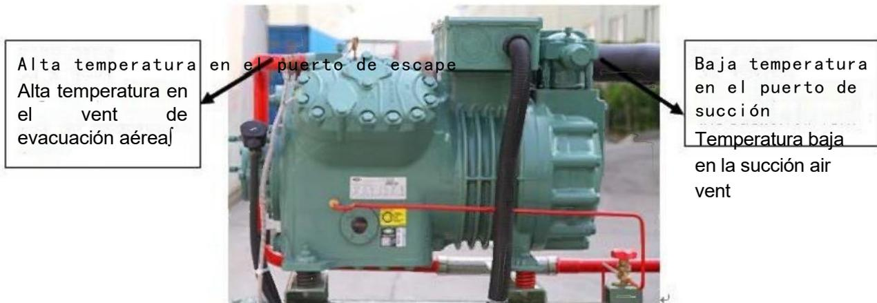
**Figura 19 Compresor Chart 19 Compressor**
