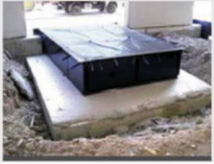
箱式基坑 Box foundation pit
