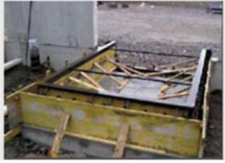
标准基坑 Standard Foundation pit
