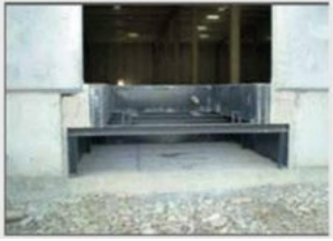
带尾板插槽钢结构预制基坑 Precasting Foundation Pit of Steel structure with Tailboard slot
